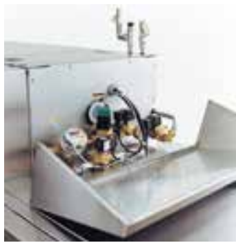
The pressure reduction valve, the magnetic valves and the final rinse water meter are placed conveniently behind a hinged door.
