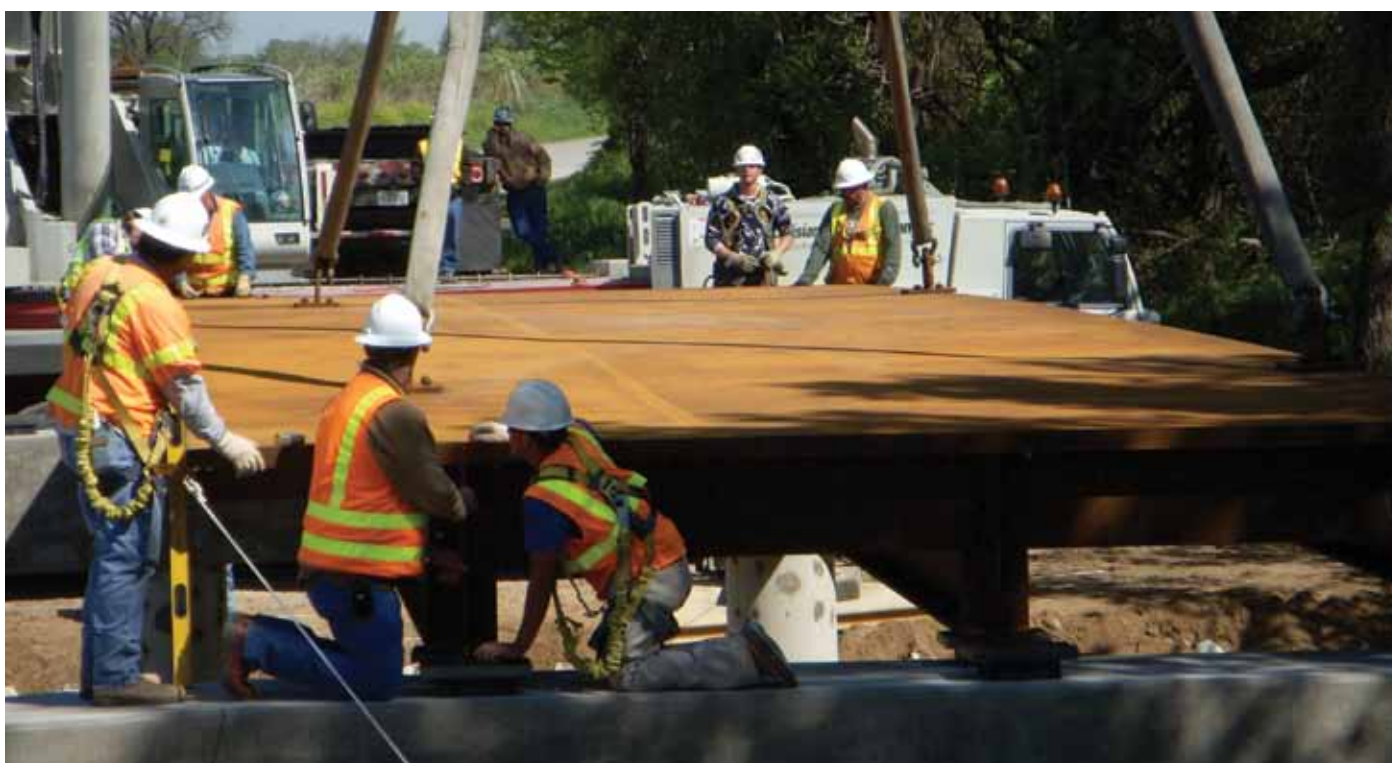
Installation of new SPS Bridge Deck
