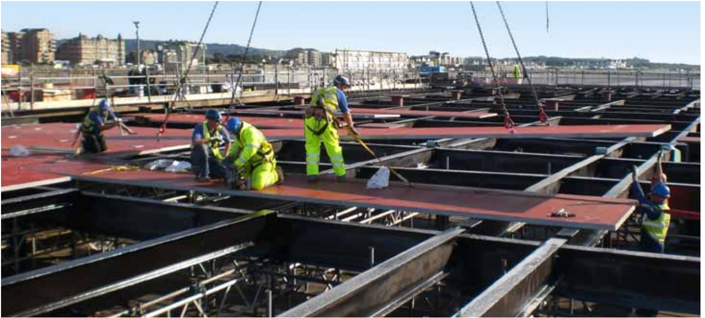
SPS Floor panels are bolted into position and can be as easily unbolted for reuse at the end of a structure's life
