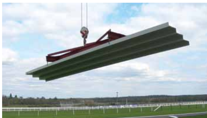
Lifting a pre-assembled triple unit of SPS Terraces
