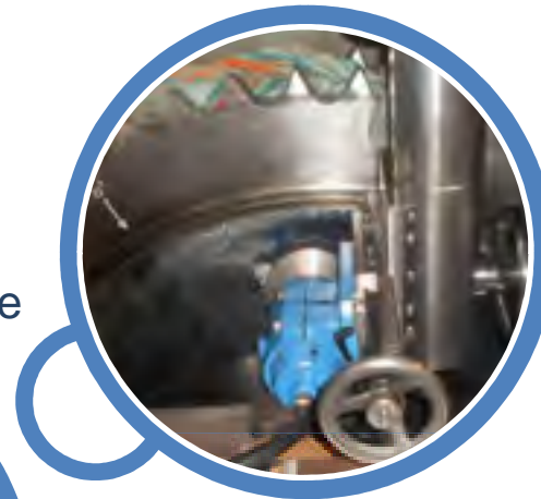
Thrust bearing repairing
